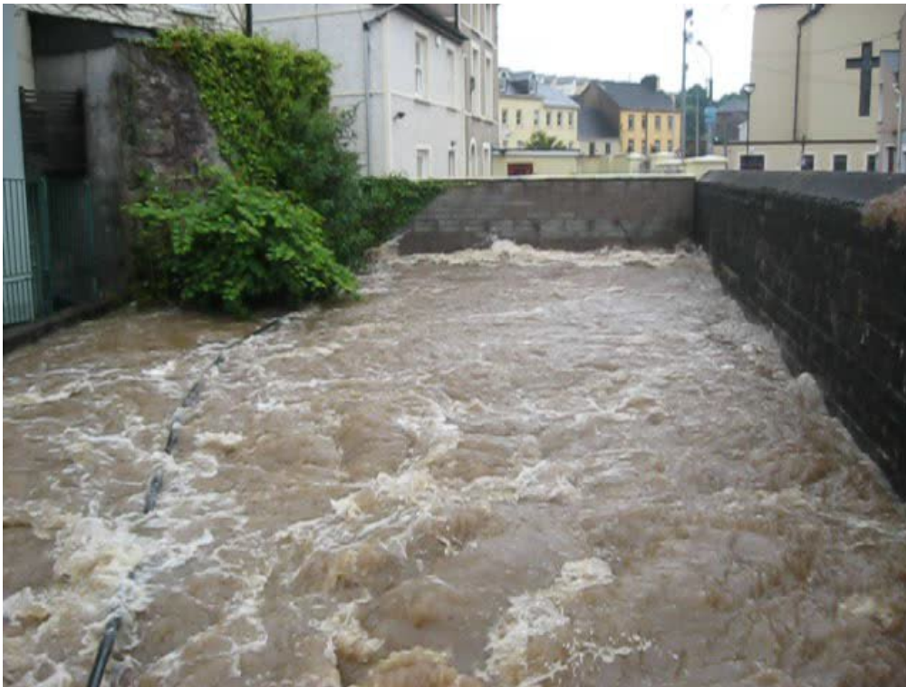
Entrance to culvert at Orchard Court. This view is a still from a video recorded at shortly after 5.00am. As with the culvert at the Church, I was advised that the flood had been observed earlier at a level of 10 blocks down from the top of the wall. See following photo.
